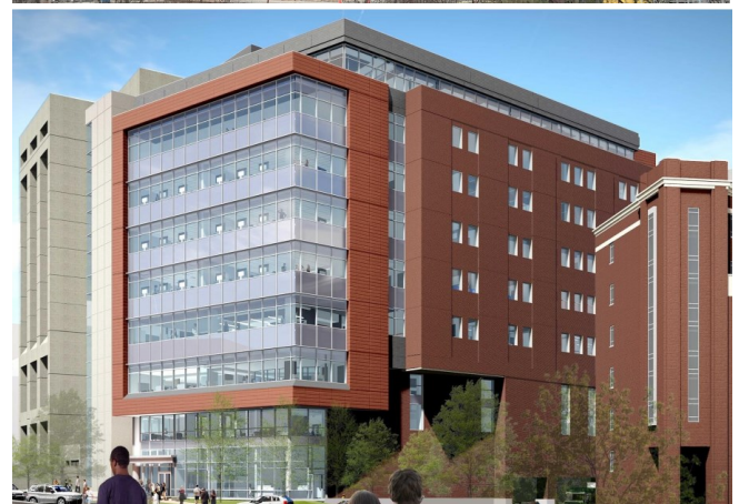
Current Construction Photo (top) and Rendering Comparison (bottom).
