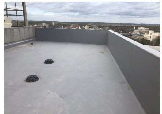
Roofing Membrane Installed at Level 8
