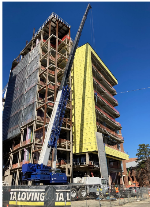
Erection of the 23,000 lb. Precast Panel
