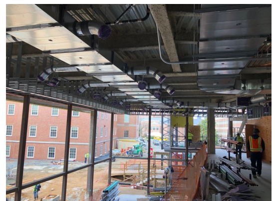
2nd Floor Interior Progression
